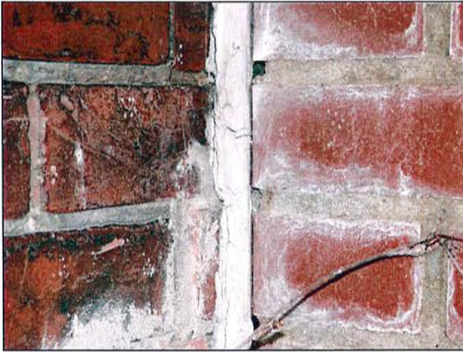
PHOTO 55: Exterior brick caulking
