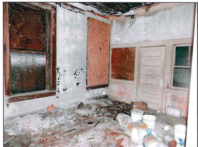
PHOTO 18: Room on 2 nd floor of east addition
