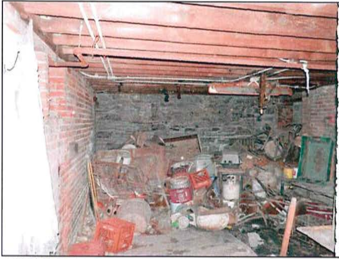
PHOTO 31: Basement room in east addition
