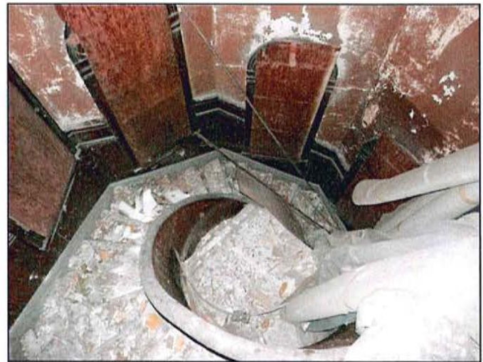
PHOTO 26: Northwest spiral stairs
