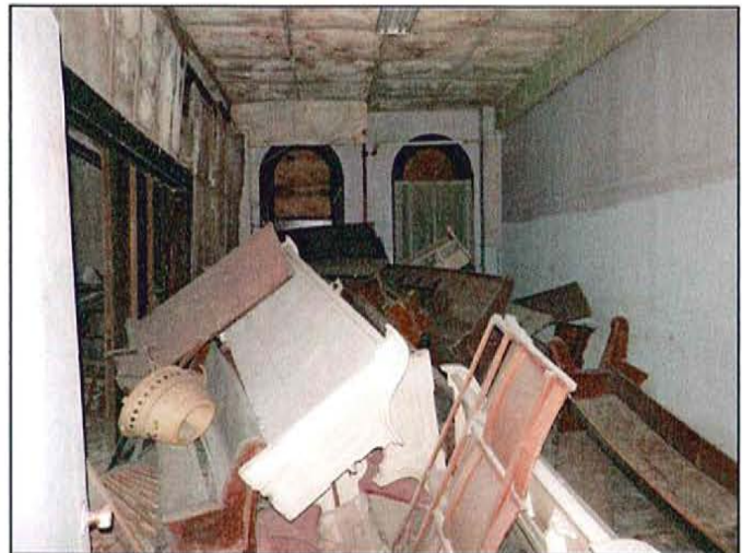
PHOTO 14: Room on 1 st floor of east addition
