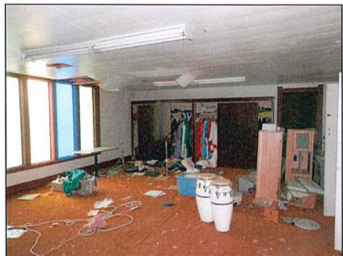
PHOTO 24: 2 nd Floor room, west side of structure
