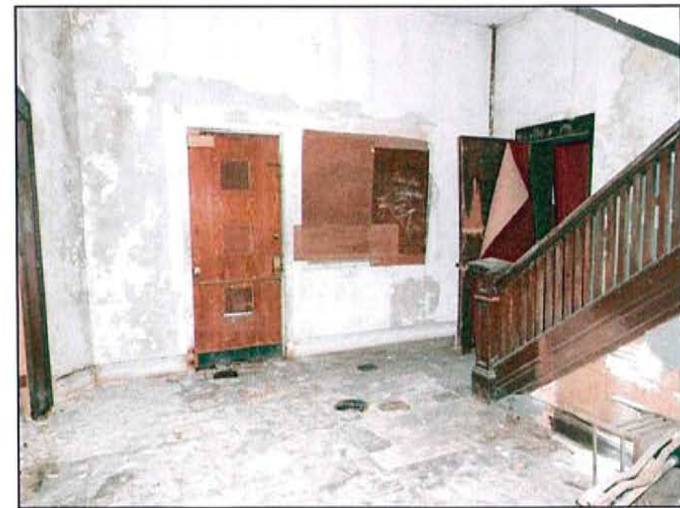
PHOTO 12: South central stair lobby (1 st floor)
