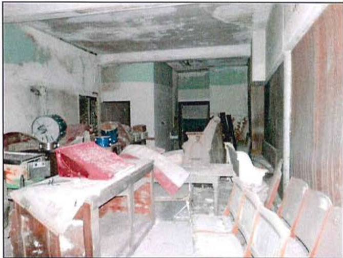
PHOTO 15: Room on 1 st floor of east addition
