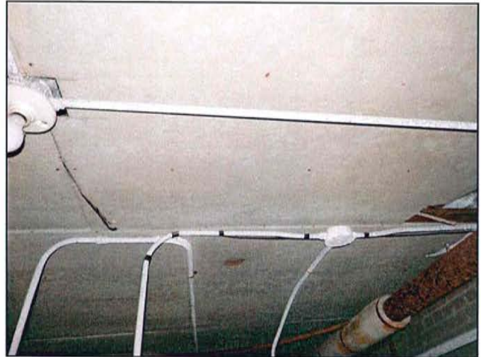
PHOTO 34: Transite ceiling in basement boiler room
