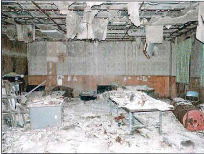
PHOTO 13: Room on 1 st floor of east addition
