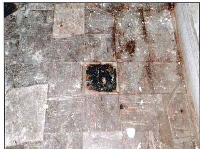
PHOTO 42: 9" x 9" Black floor tile in east addition
