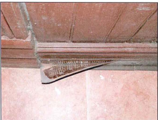
PHOTO 53: Cove base and mastic
