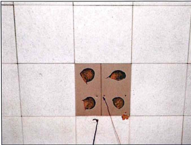
PHOTO 43: 1' x 1' Ceiling tile with adhesive pucks
