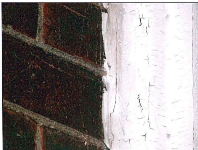
PHOTO 59: Exterior window caulking
