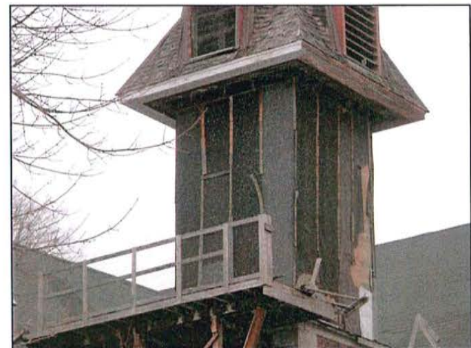
PHOTO 60: Roofing shingle on west structure section
