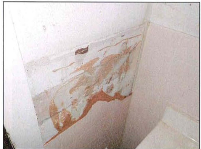
PHOTO 52: Wall board mastic
