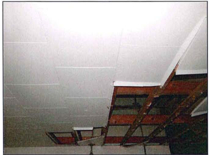
PHOTO 44: 1' x 1' ceiling tile (stapled)
