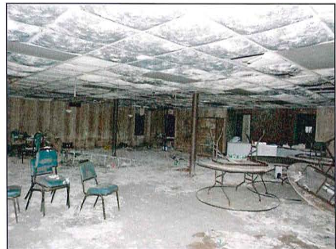
PHOTO 28: Meeting hall in basement
