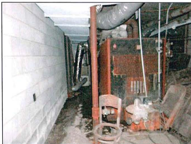
PHOTO 29: Basement boiler room
