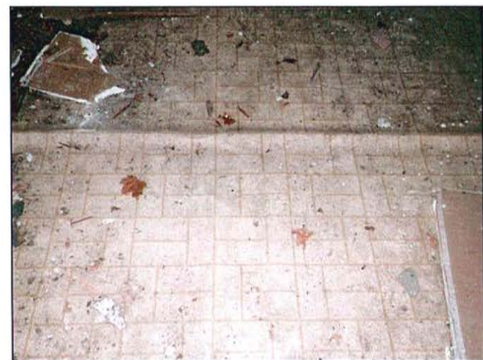
PHOTO 48: Tan brick pattern linoleum
