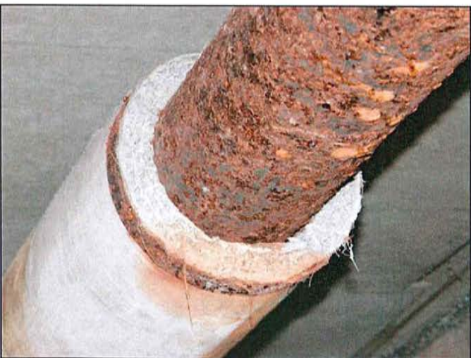
PHOTO 35: Aircell-type pipe insulation in basement
