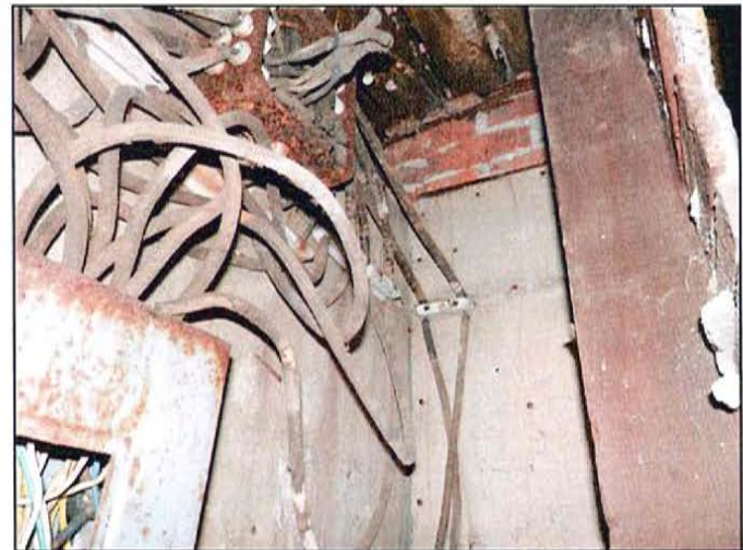
PHOTO 40: Insulating board in 1 st floor electrical closet
