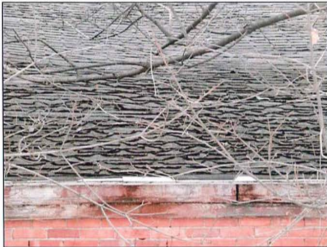
PHOTO 57: Roofing shingle on east addition
