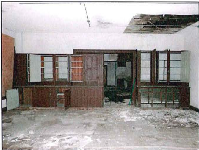
PHOTO 17: Room on 2 nd floor of east addition
