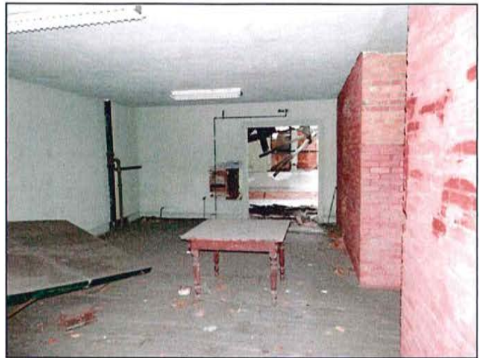
PHOTO 20: Room on 3 rd floor of east addition
