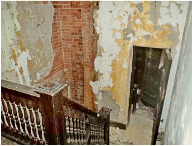
Figure 7- damage at Stair 106 at east side of Organ from roof leak.
