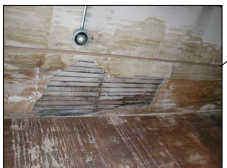
CLG & WALL WATER DAMAGE
