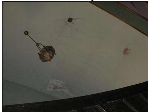
WATER DAMAGE MAIN CEILING
