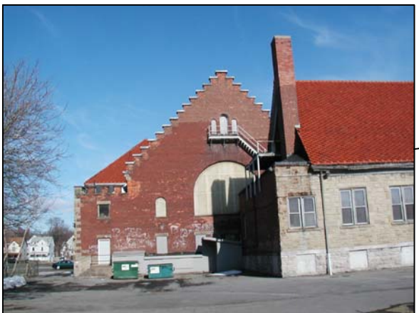
WATER DAMAGE AT BRICK ALONG GABLE STEPS
