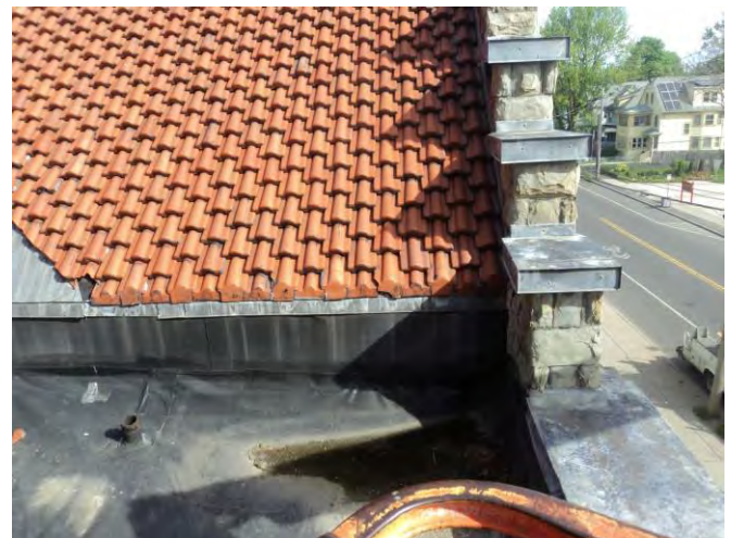
Fig 3 –NW flat roof area; undersized roof drain
