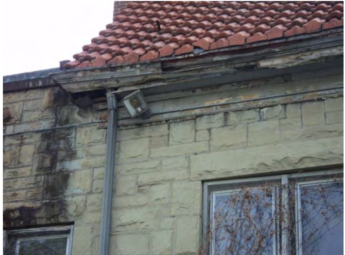
Figure 8- deteriorated wood eave and gutter system at westside of Chapel.
