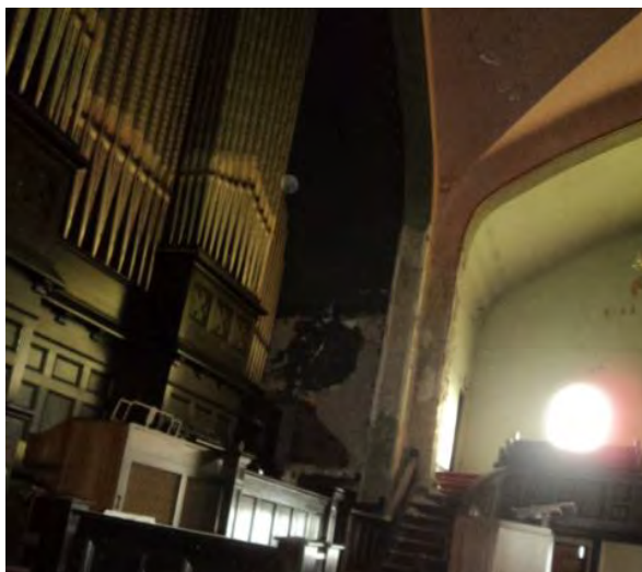
Figure 5 – Organ area with water damage
