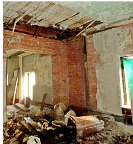
Fig 4 – Vest Rm 107 – damage from roof leak
