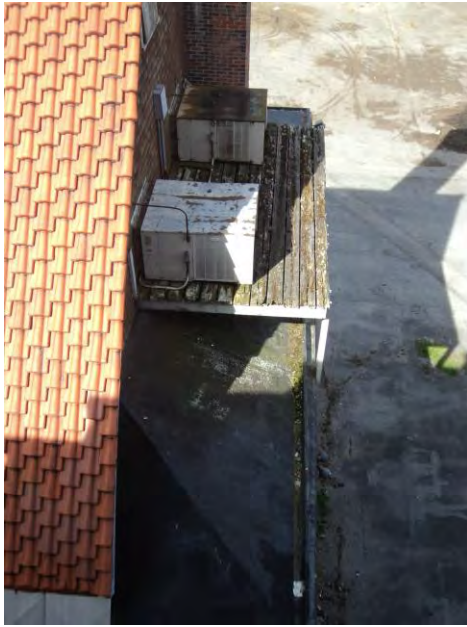
Fig 7 - Platform over hipped coated metal roof at northside of Chapel
