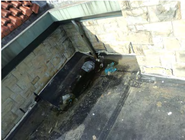
Figure 1 – Northeast flat roof area ; undersized roof drain; improper membrane installation.
