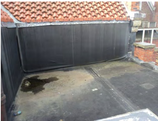
Figure 4 – Southeast flat roof; membrane wrinkles
