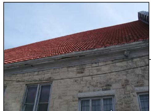
SOFFITS & FASCIA DETERIORATED
