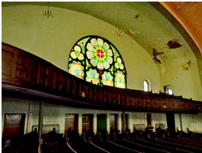
Fig 3 –NW Balcony Area; ceiling damage.
